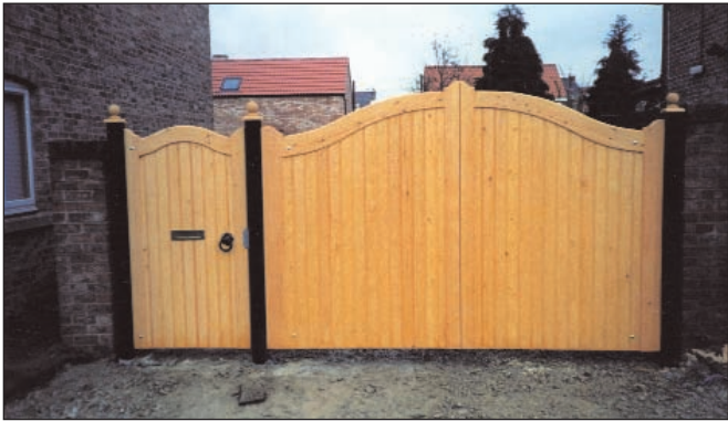
Bow-shaped top framed brace & ledge
