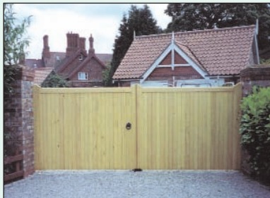
Straight top frame brace & ledge
